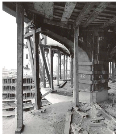
Figure 3: ring beam and haunch detail at perimeter columns, Marina City towers [drawing done later by author]
