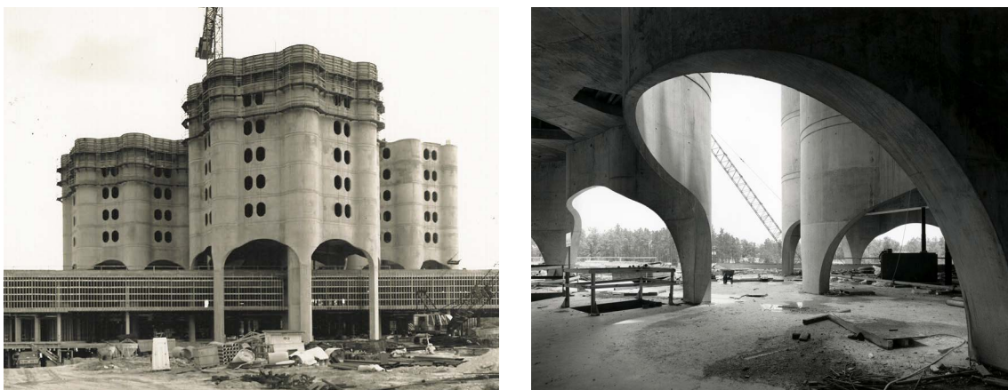
Figures 23, 24: Providence Hospital, Mobile, AL, Bertrand Goldberg Associates, 1986
